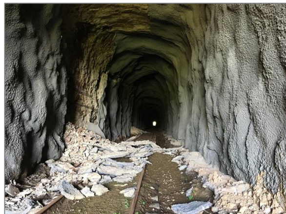
Photograph 6-26. Interior of Walcott Tunnel
