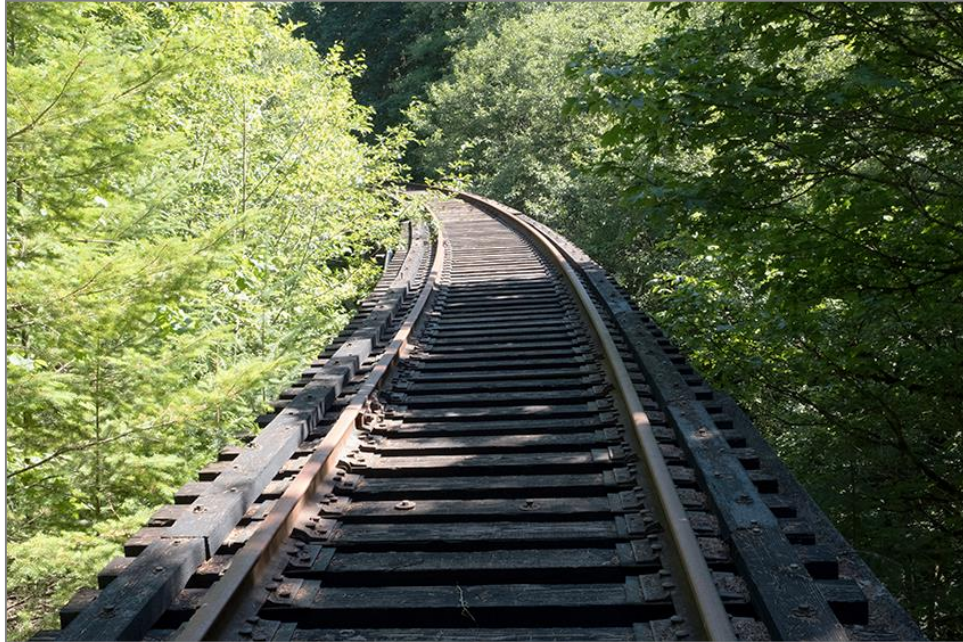
Photograph 6-35. Camp Creek Trestle
