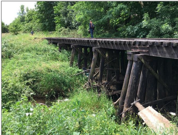
Photograph 6-36. Trestle across West Fork Dairy Creek
