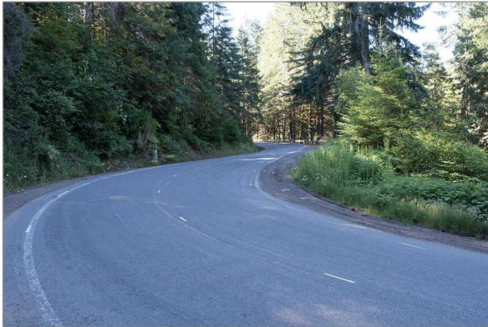
Photograph 6-28. NW Timber Road
