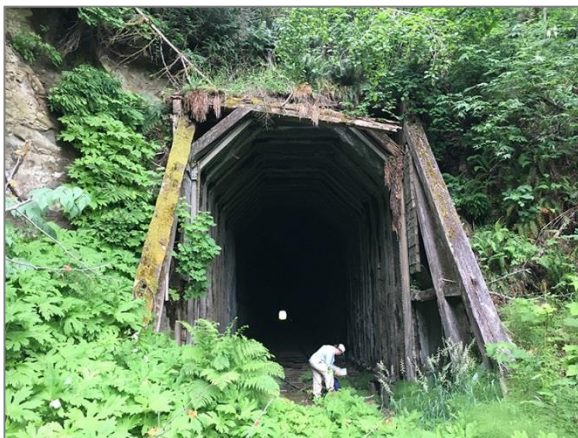
Photograph 6-25. East entrance to Walcott Tunnel
