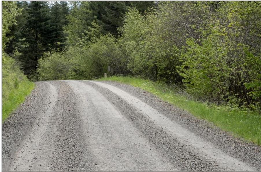
Photograph 6-29. NW Strassel Road
