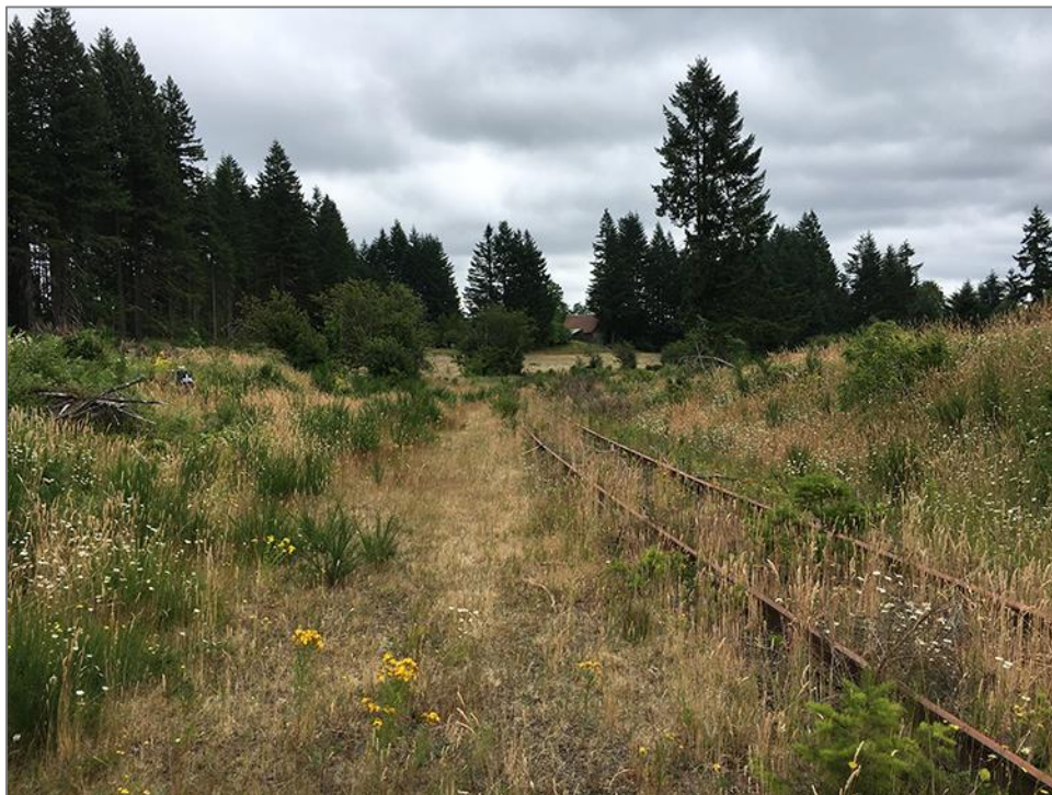
Photograph 6-8. Relatively clear areas near Scofield crossing
