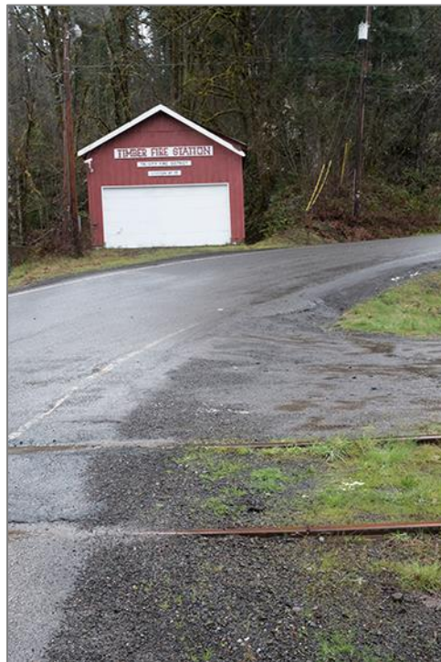
Photograph 6-10. Historic Timber Fire Station
