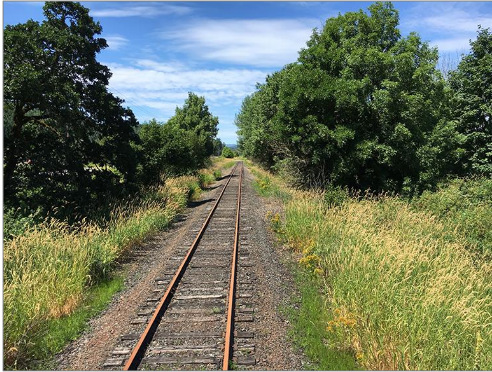
Photograph 6-2. Only extended clear section of rail (near Banks)
