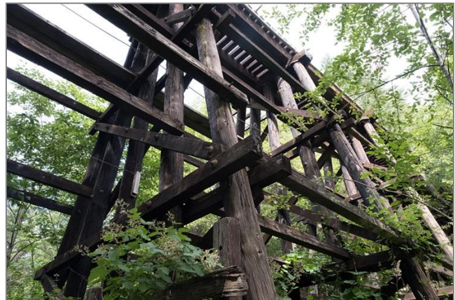
Photographs 6-23 and 6-24. Williams Creek Trestle
